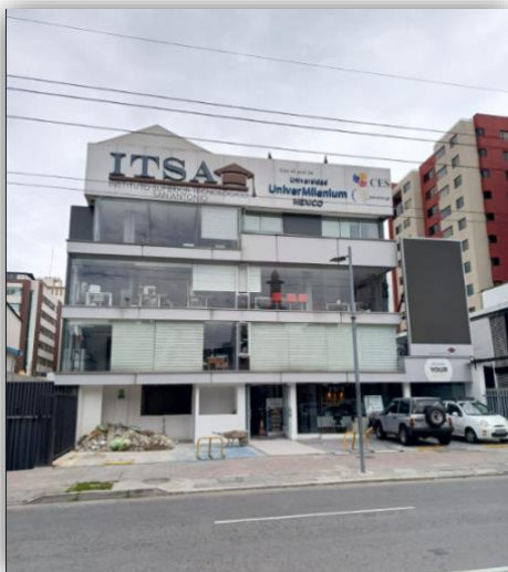
Fachada Instituto ITSA
